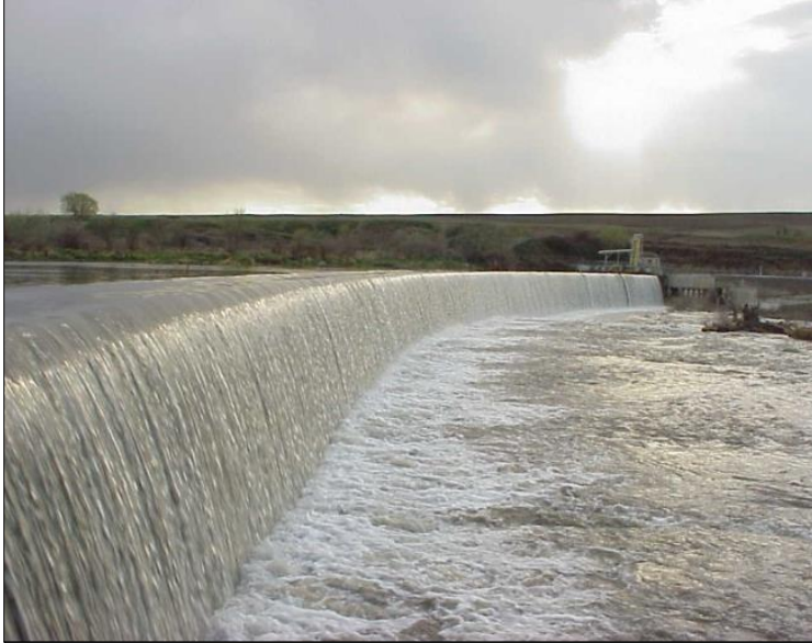
Three Mile Falls Dam, 1998
